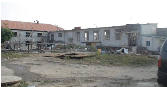
Own campus of UAO in construction (2005)
